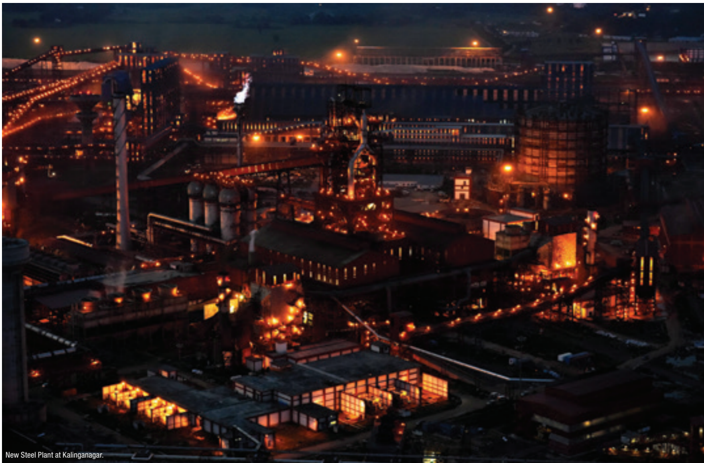
New Steel Plant at Kalinganagar.
